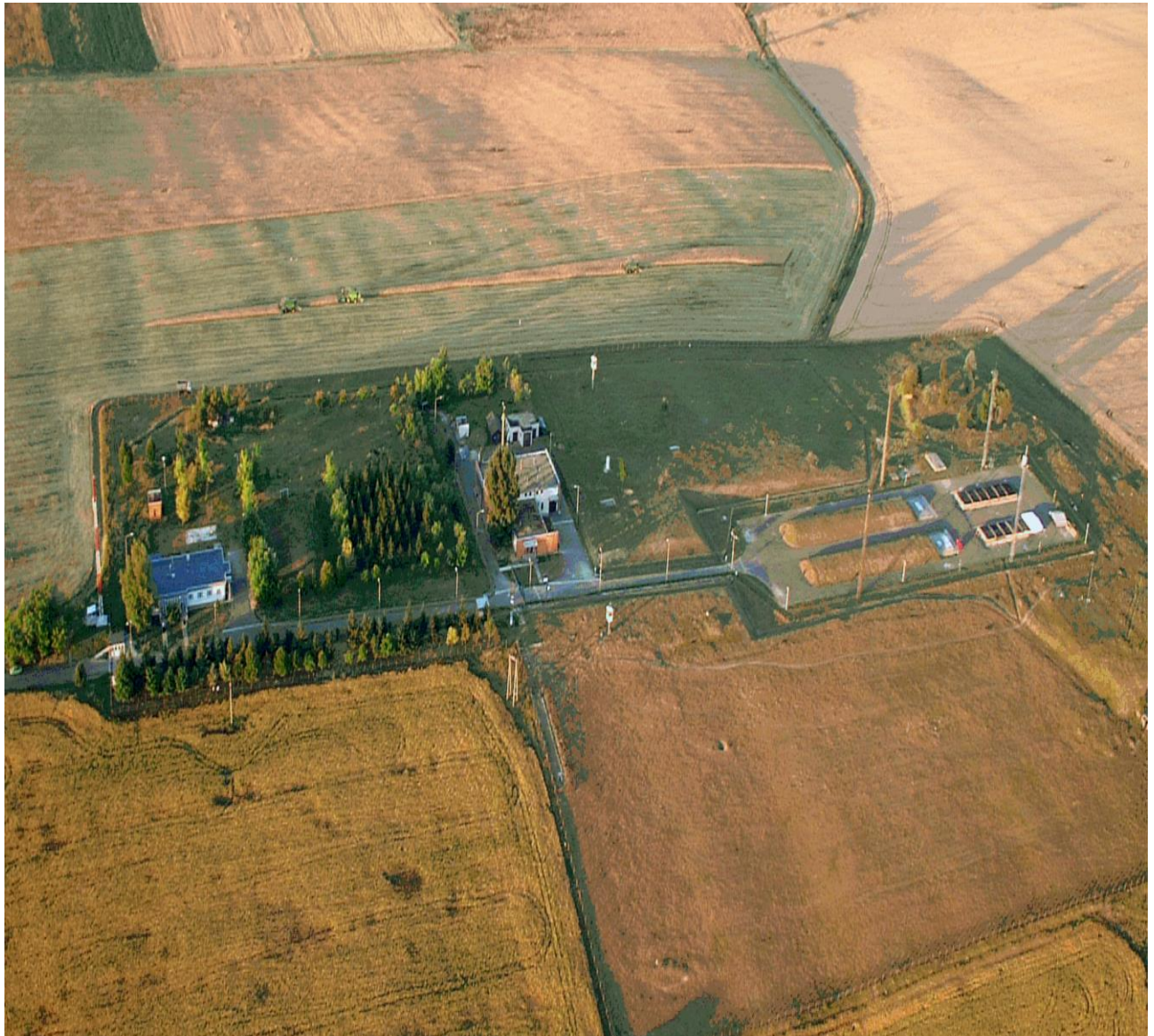
Figure 2.6-1: Bird view of the Radioactive Waste Treatment and Disposal Facility (Source: http://www.rhk.hu/images/sajto/rhft-madartavlat.jpg )
