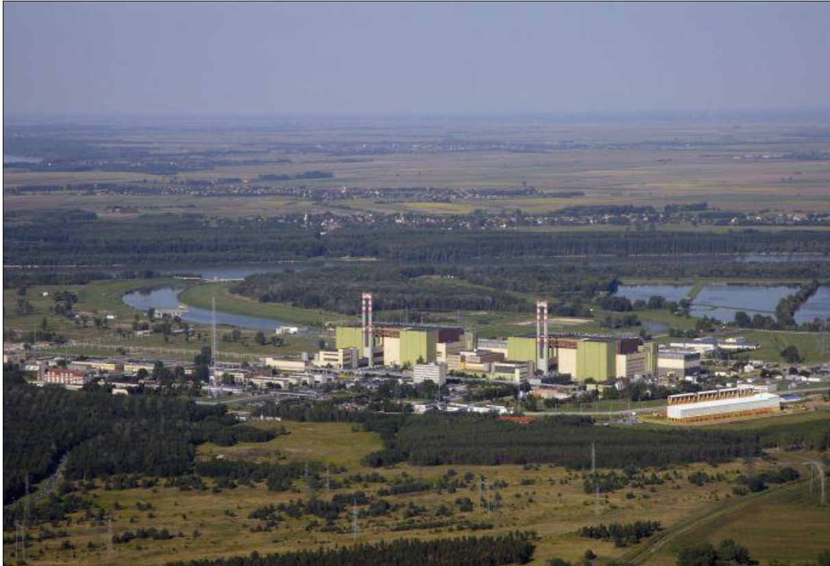
Paks Nuclear Power Plant (Source: www.atomeromu.hu )
