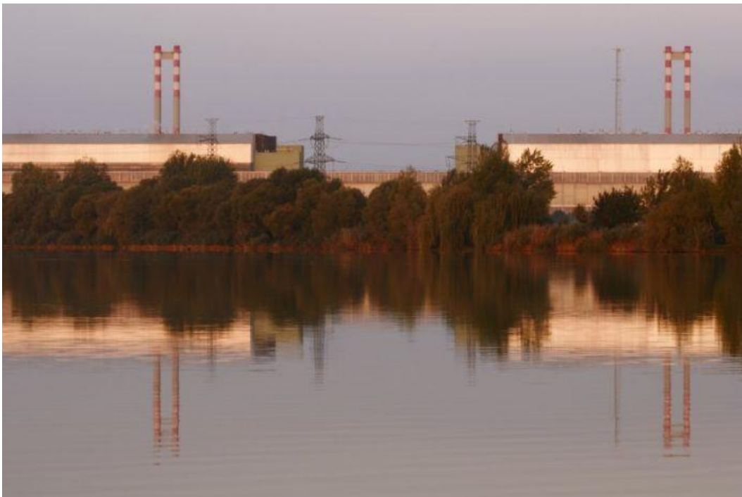
Figure 2.1-1: View of Paks Nuclear Power Plant (Source: www.atomeromu.hu )
