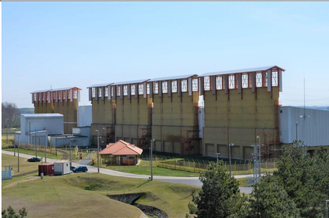
Spent Fuel Interim Storage Facility (Source: https://rhk.hu/gallery/a-kiegett-kazettak-atmeneti-tarolojakkat/files )
